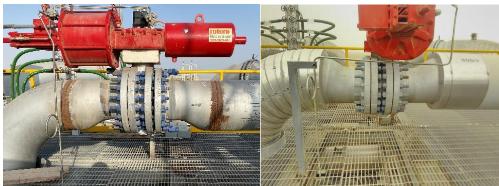
Figure 1 – Example of a “punch-list” item discovered late in the EPC process. The amine acid gas line needs to be free draining towards the left. Note solution required cutting & re-welding numerous pipe sections, removing and reinstalling insulation, remounting valve actuator for clearance as well as re-routing electrical and instrument air connections. This facility had 3 trains with identical installations on each train. Issue was discovered after piping in several of the trains had already been insulated.
