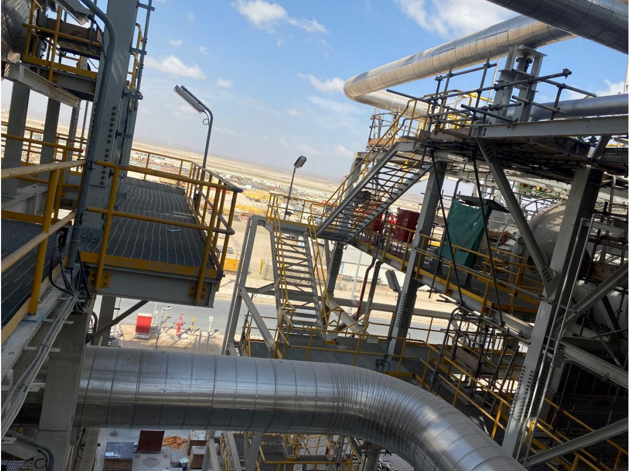
Figure 2 - Reaction Furnace structure separate from Claus Reactor/Condenser structure. Combining/connecting these two structures potentially would have reduced construction quantities as well as saved operations staff the need to repeatedly climb up and down numerous stair towers.
